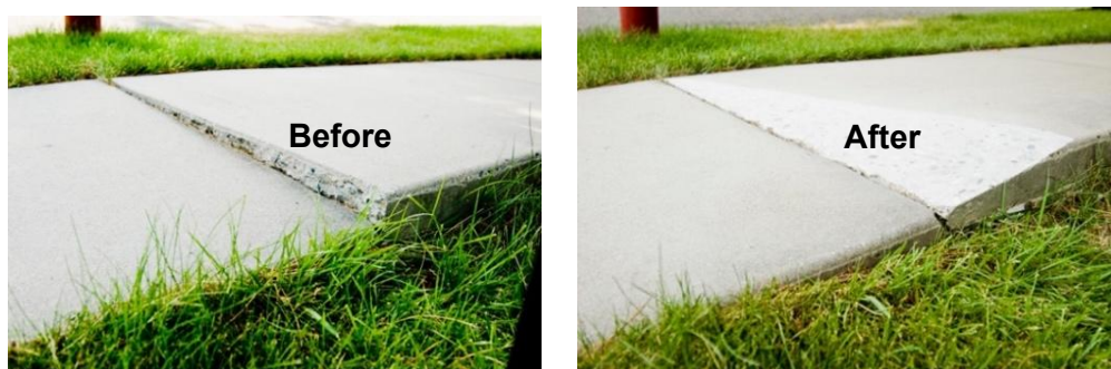
Figure 7: Precision Sidewalk Safety Work Example
